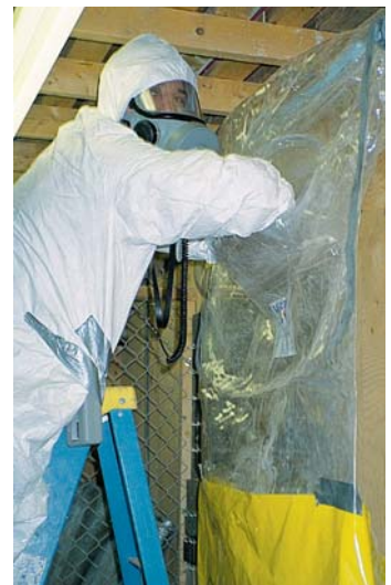
LINDSAY ASBESTOS REMOVAL
