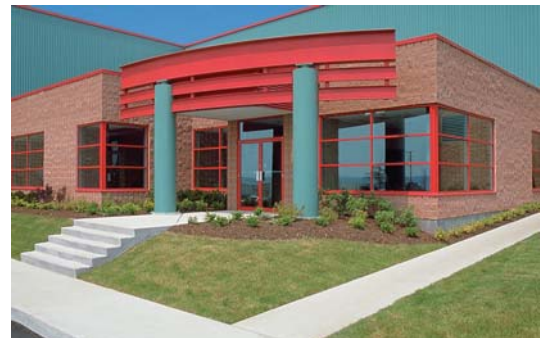
LEROUX STEEL BURNSIDE INDUSTRIAL PARK; DARTMOUTH, NOVA SCOTIA
