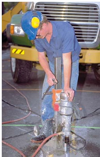
LINDSAY CONCRETE CORING
