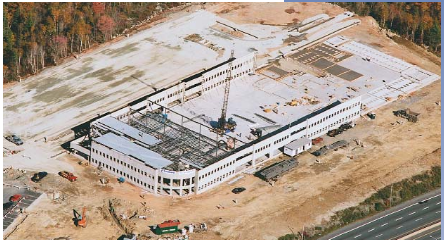
ABOVE: Atboro House in Burnside Industrial Park is comprised of 60 tilt-up concrete wall panels, standing up to 29 feet high and 34 feet wide and weighing up to 80,000 pounds.
