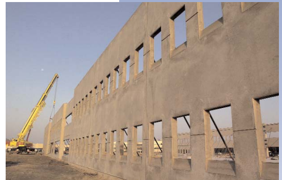
ABOVE: Atboro House in Burnside Industrial Park is comprised of 60 tilt-up concrete wall panels, standing up to 29 feet high and 34 feet wide and weighing up to 80,000 pounds.
