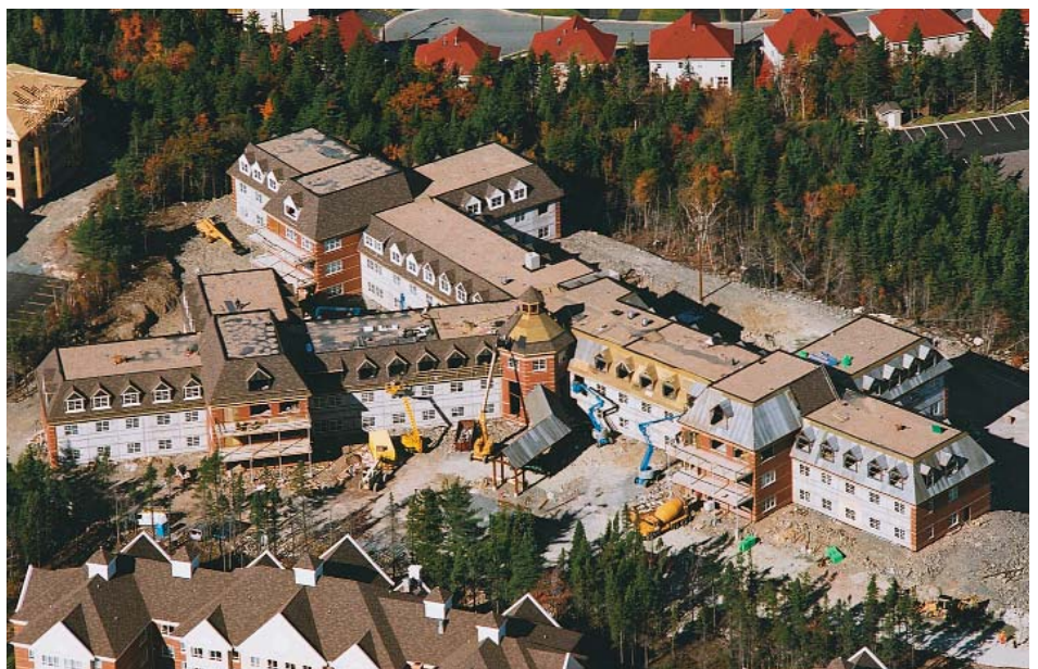
RIGHT: Shannex Quality Living, a 180-bed nursing home in the Clayton Park area, is an example of the diverse uses of Lindsay tilt-up.
