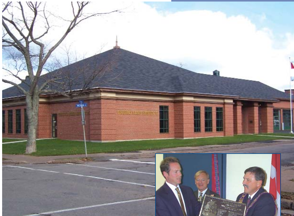
ABOVE: the newly constructed fire station in Truro, Nova Scotia gives the town's firefighters a modern new facility that blends seamlessly with the neighborhood's historical buildings.
