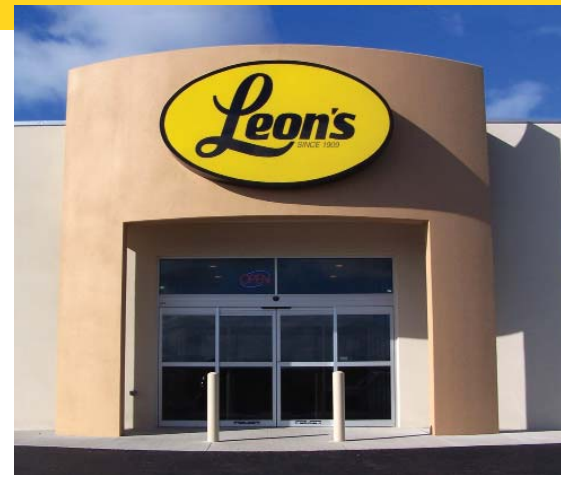
Leon's new store in the Truro Power Centre boasts a clean, simple design using tilt-up panels.
