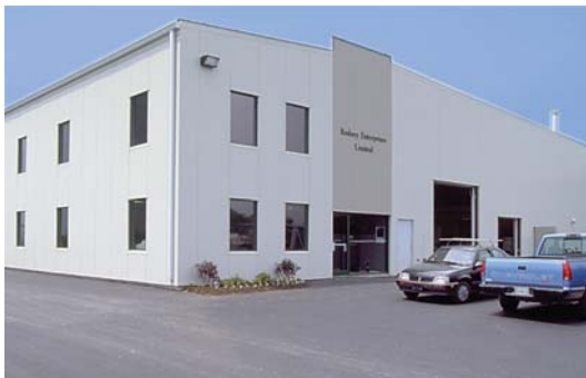
RODNEY ENTERPRISES LIMITED BURNSIDE INDUSTRIAL PARK; DARTMOUTH, NOVA SCOTIA
