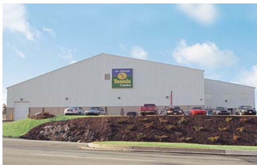
AIR ATLANTIC TENNIS CENTRE BAYERS LAKE INDUSTRIAL PARK; HALIFAX, NOVA SCOTIA
