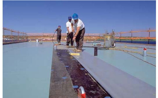
CASINO NOVA SCOTIA HOTEL ROOFING IN PROGRESS HALIFAX, NOVA SCOTIA
