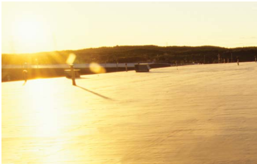
FINISHED FLEECEBACK ROOF 18 TOPPLE DRIVE; DARTMOUTH, NOVA SCOTIA
