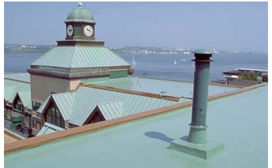
CASINO NOVA SCOTIA HOTEL FINISHED ROOF HALIFAX, NOVA SCOTIA
