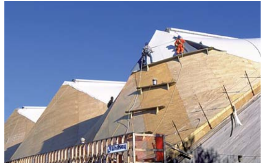
DALHOUSIE MEMORIAL ARENA ROOFING IN PROGRESS HALIFAX, NOVA SCOTIA
