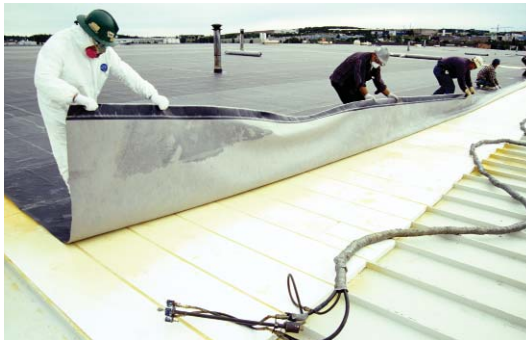
APPLICATION OF CARLISLE FAST 100 FLEECEBACK ROOFING 18 TOPPLE DRIVE; DARTMOUTH, NOVA SCOTIA
