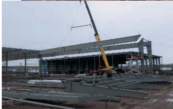
ABOVE: The second installment nears completion, using a 65-tonne crane.
