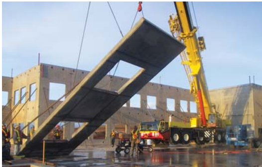
TILT-UP PANEL ERECTION AT WINDSOR HIGH SCHOOL WINDSOR, NOVA SCOTIA
