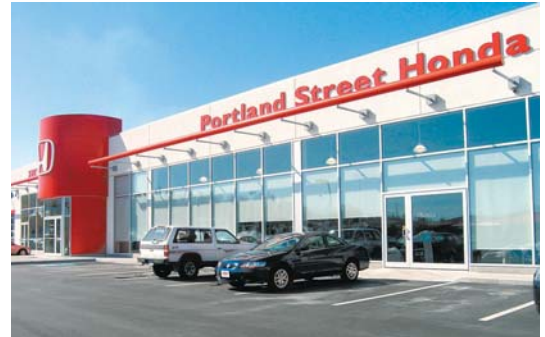
PORTLAND STREET HONDA PORTLAND STREET; DARTMOUTH, NOVA SCOTIA
