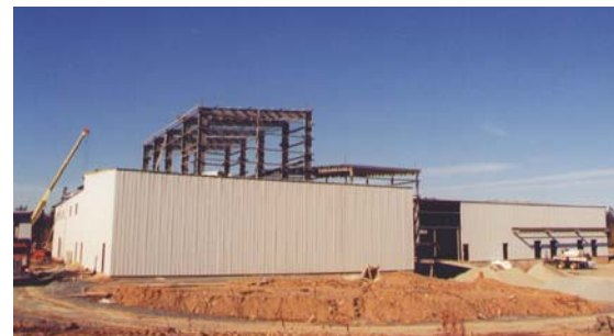
TOP: A pre-engineered metal building from American Buildings will house the Halifax Herald's new cutting edge press.
