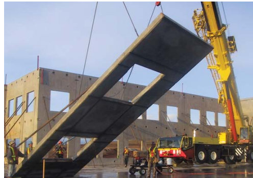
The new Windsor-West Hants high school boasts 120 tilt-up concrete panels.
