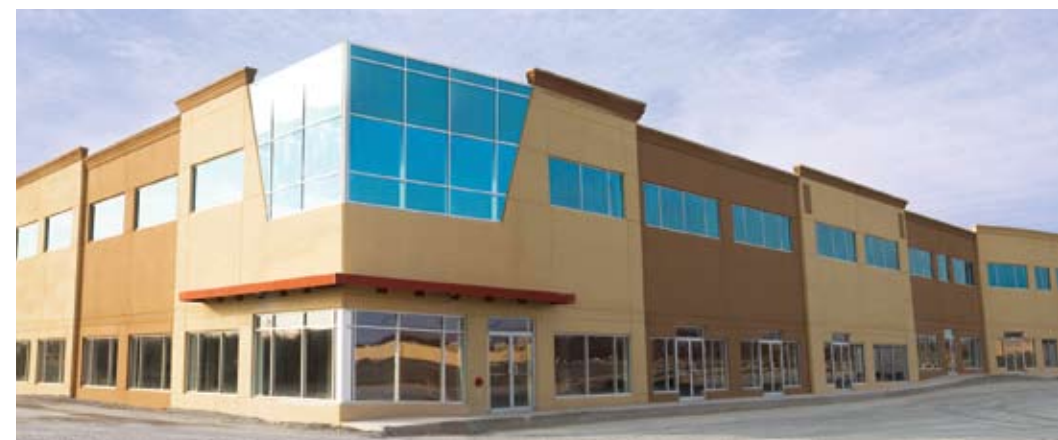
RIGHT: The 80,000 square foot retail/office building is situated at the gateway to the Bedford Commons retail development
